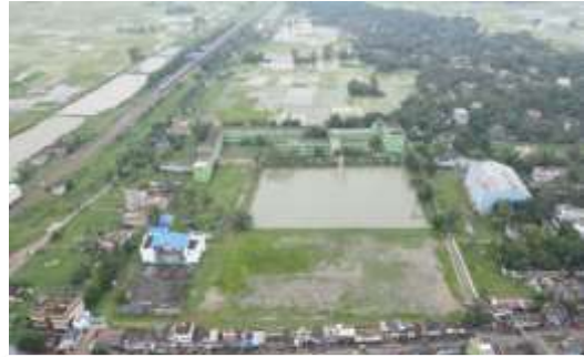
Aerial Views of the Structural area
