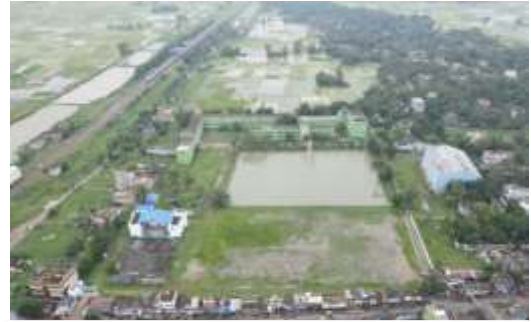
Aerial Views of the Structural area
